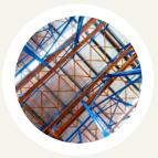
Cross Bracing are installed to the rear and top of the drive-in rack system for ultimate stability.
